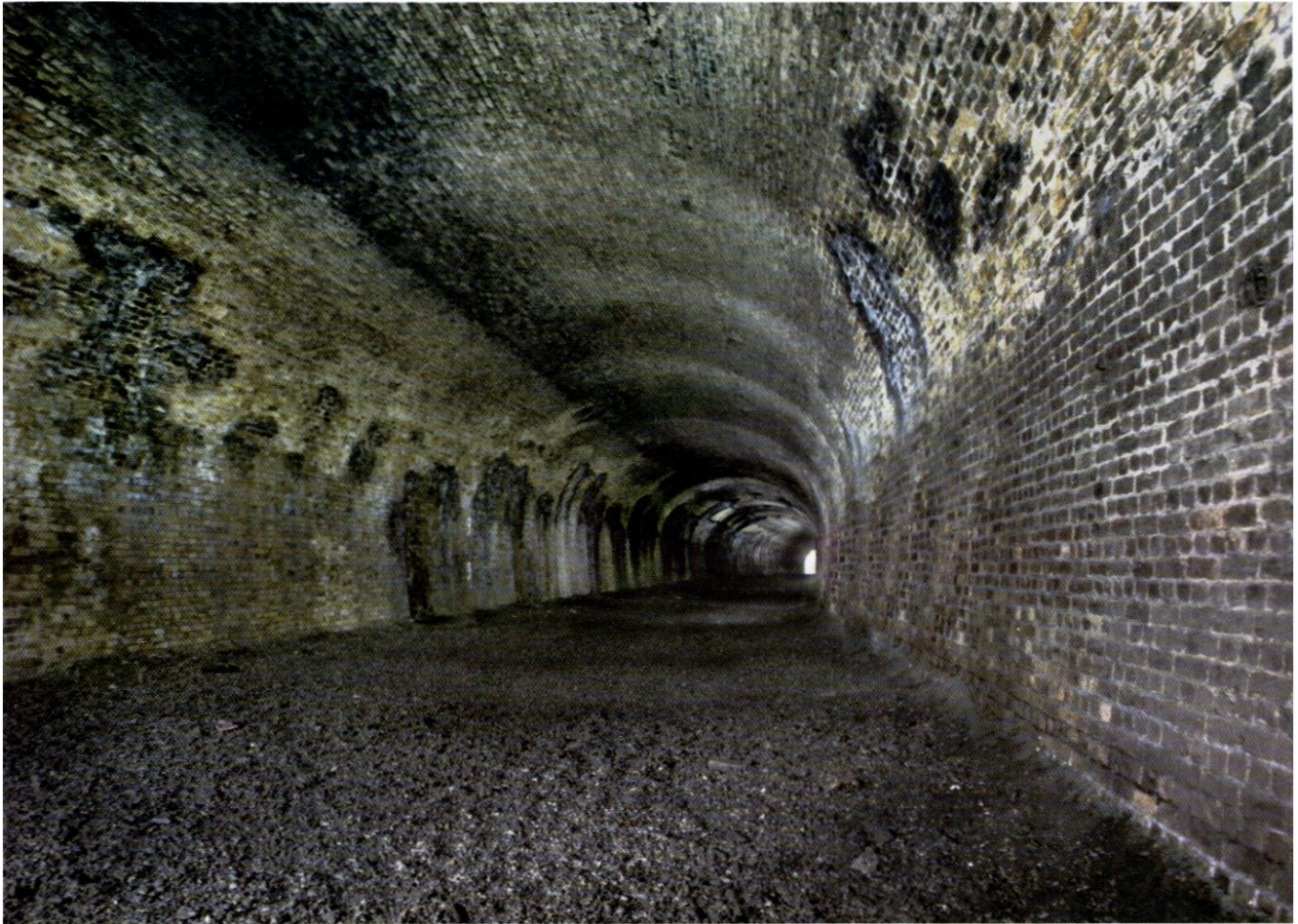
Bourne Park tunnel in 1998. The low profile of this cut-and-cover tunnel is clearly seen. Photo Nick Catford
